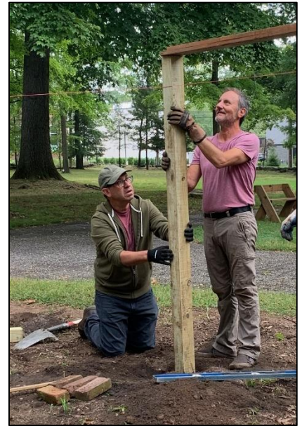
Scott Japko (2022) and Dan Coviello (2024) installing fence posts.
