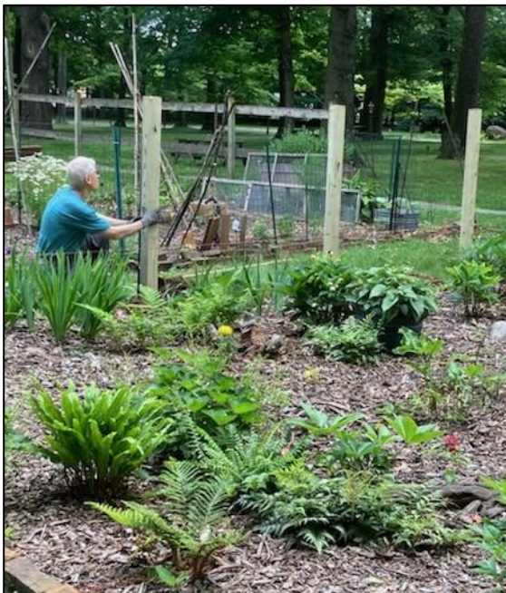
Ed Drennan (2019) was definitely hard at work installing fence posts early in the season.
